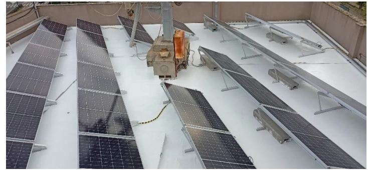
High reflective coating can boost energy production of photovoltaic panels
