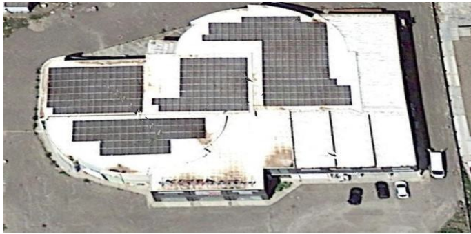
High reflective coating can boost energy production of photovoltaic panels
